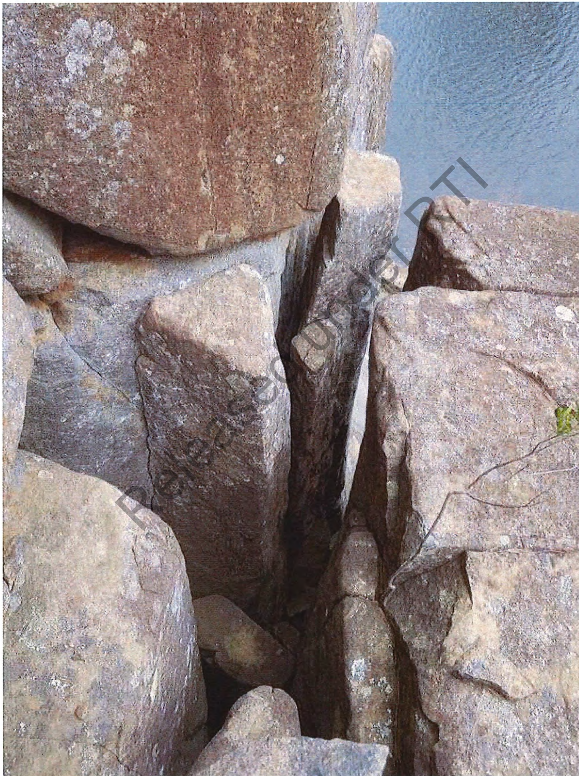
Figure 10: Open defects lower down buttress (restrained boulder is above boulder in upper left of photo)
