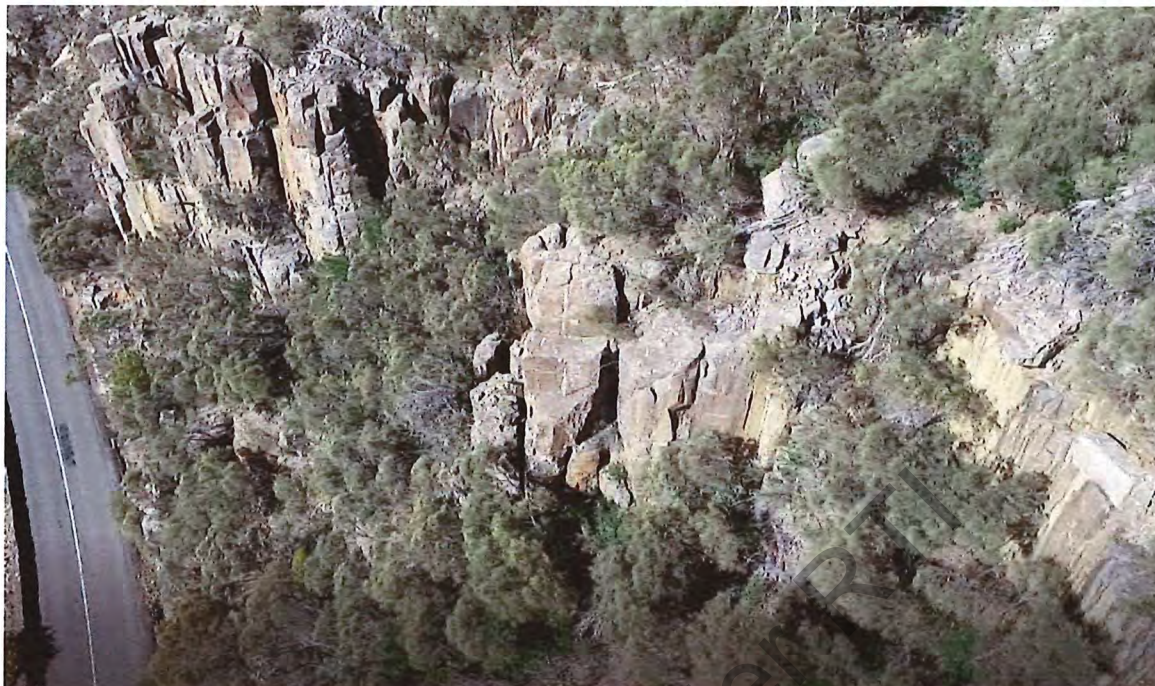
Figure 6: Buttress of interest back left; second buttress middle ground. More open cracking at top.
