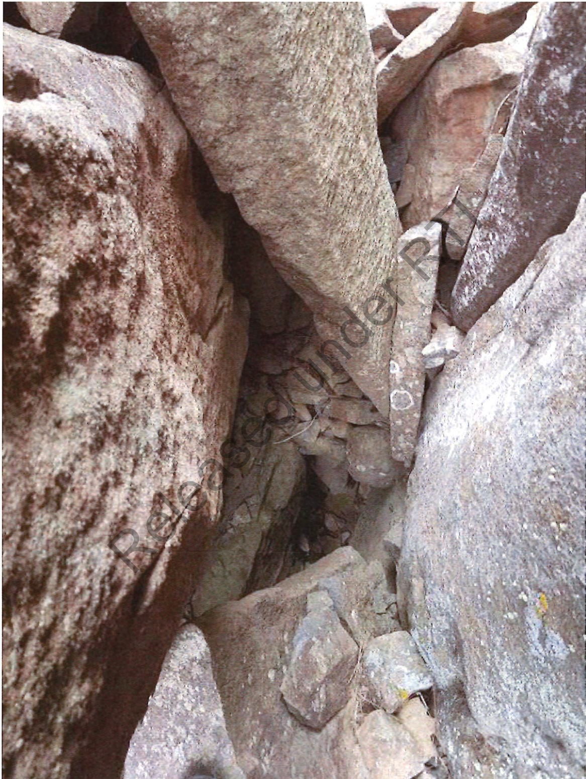
Figure 9: View from within the crack; taken a little below the base of the restrained boulder
