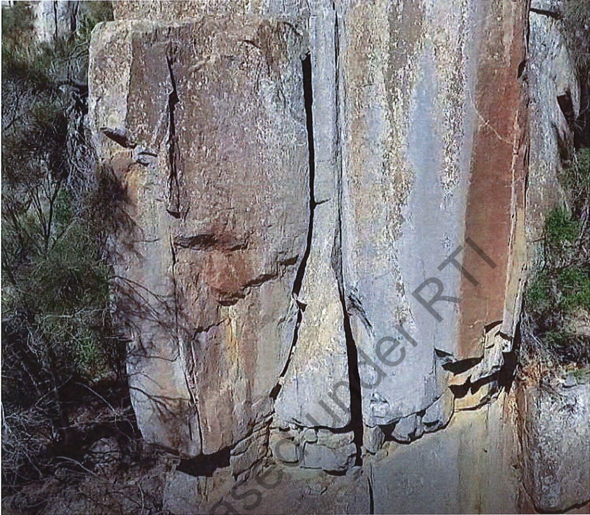
Figure 2: Undercut column with curving defect behind and crushed rock beneath
