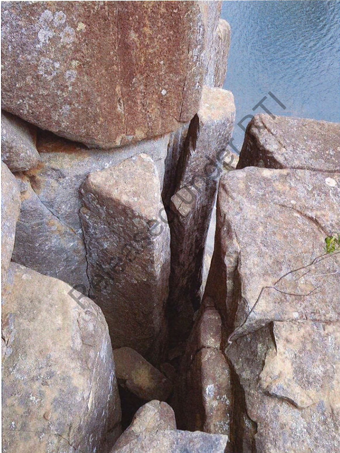
Figure 4: Open defects lower down buttress (restrained boulder is above boulder in upper left of photo)
