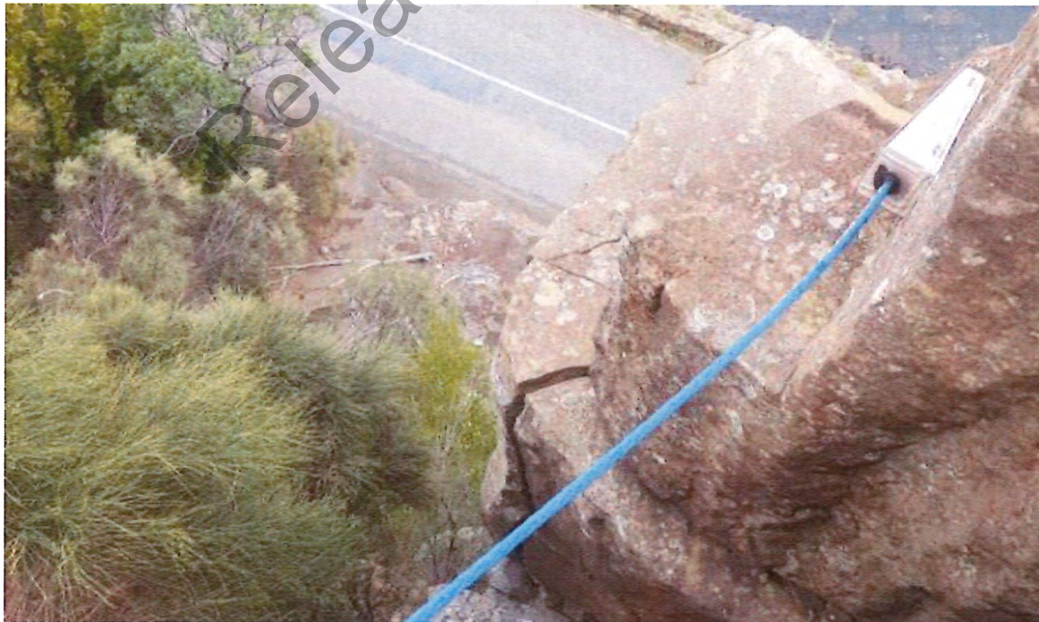
Figure 6: View of end of restraining wire on western side of boulder
