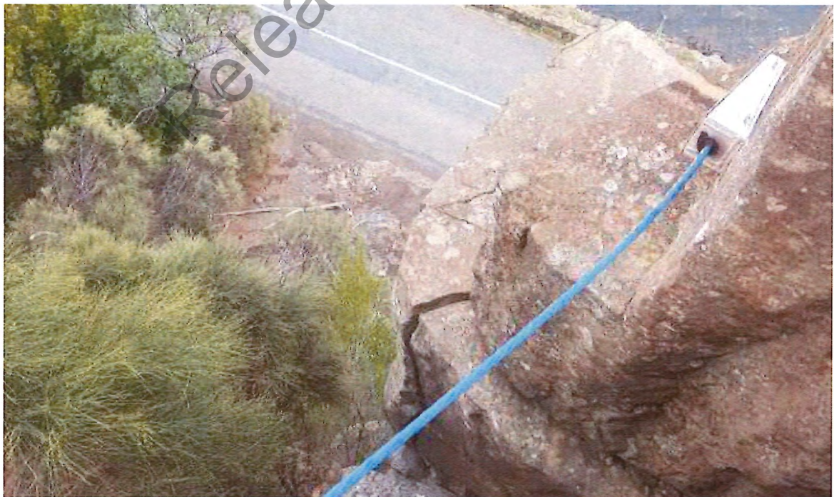
Figure 12: View of end of restraining wire on western side of boulder
