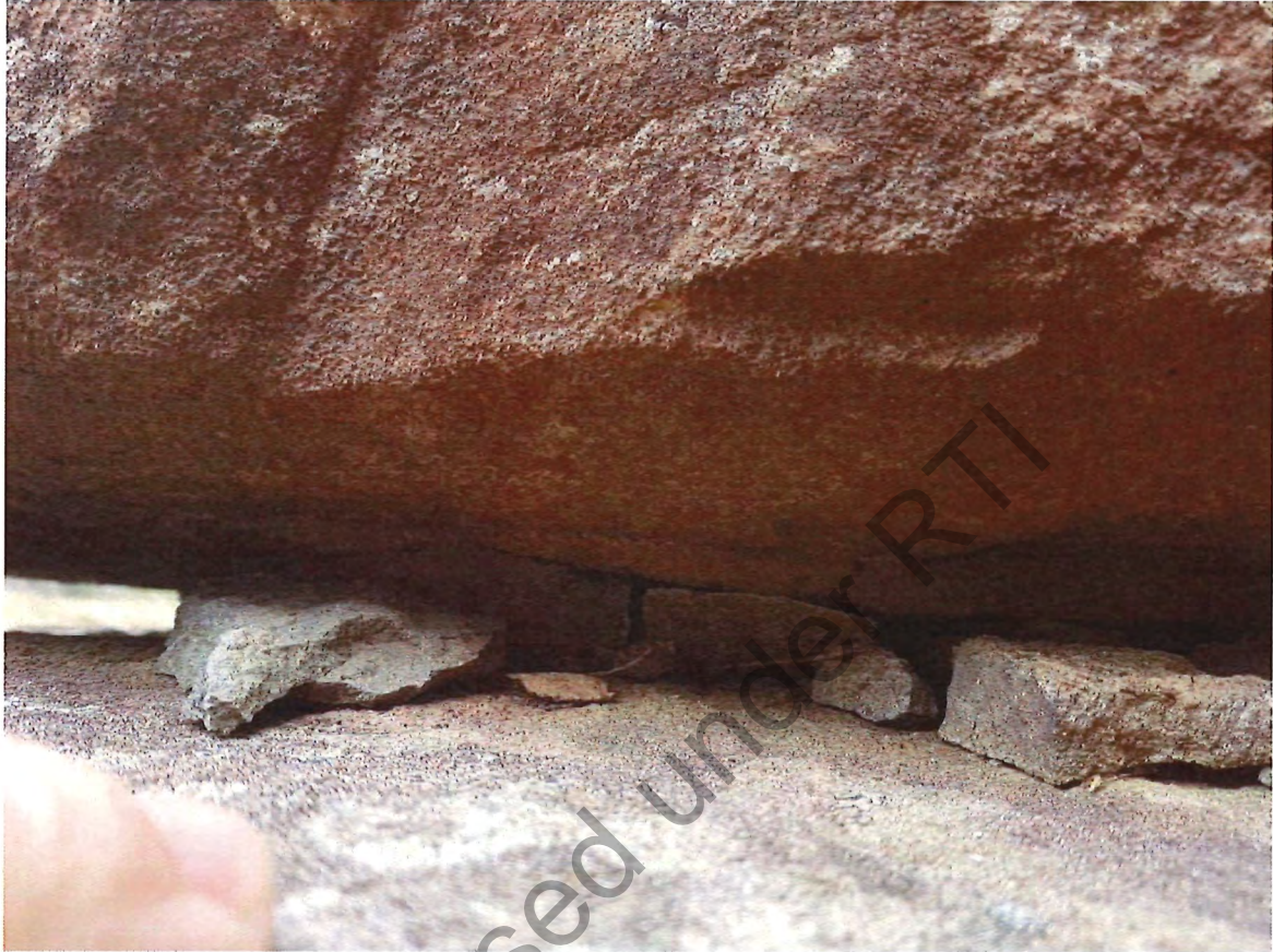
Figure 11: View under restrained boulder
