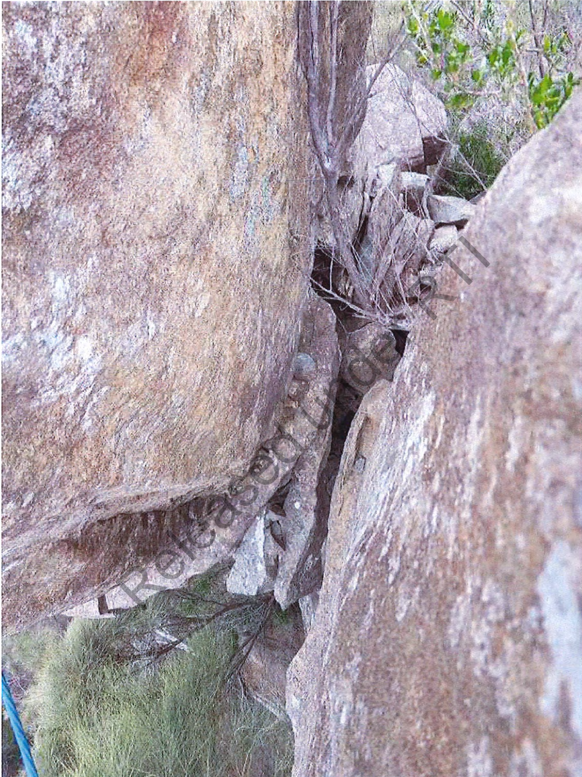
Figure 8: View down crack at back of restrained boulder
