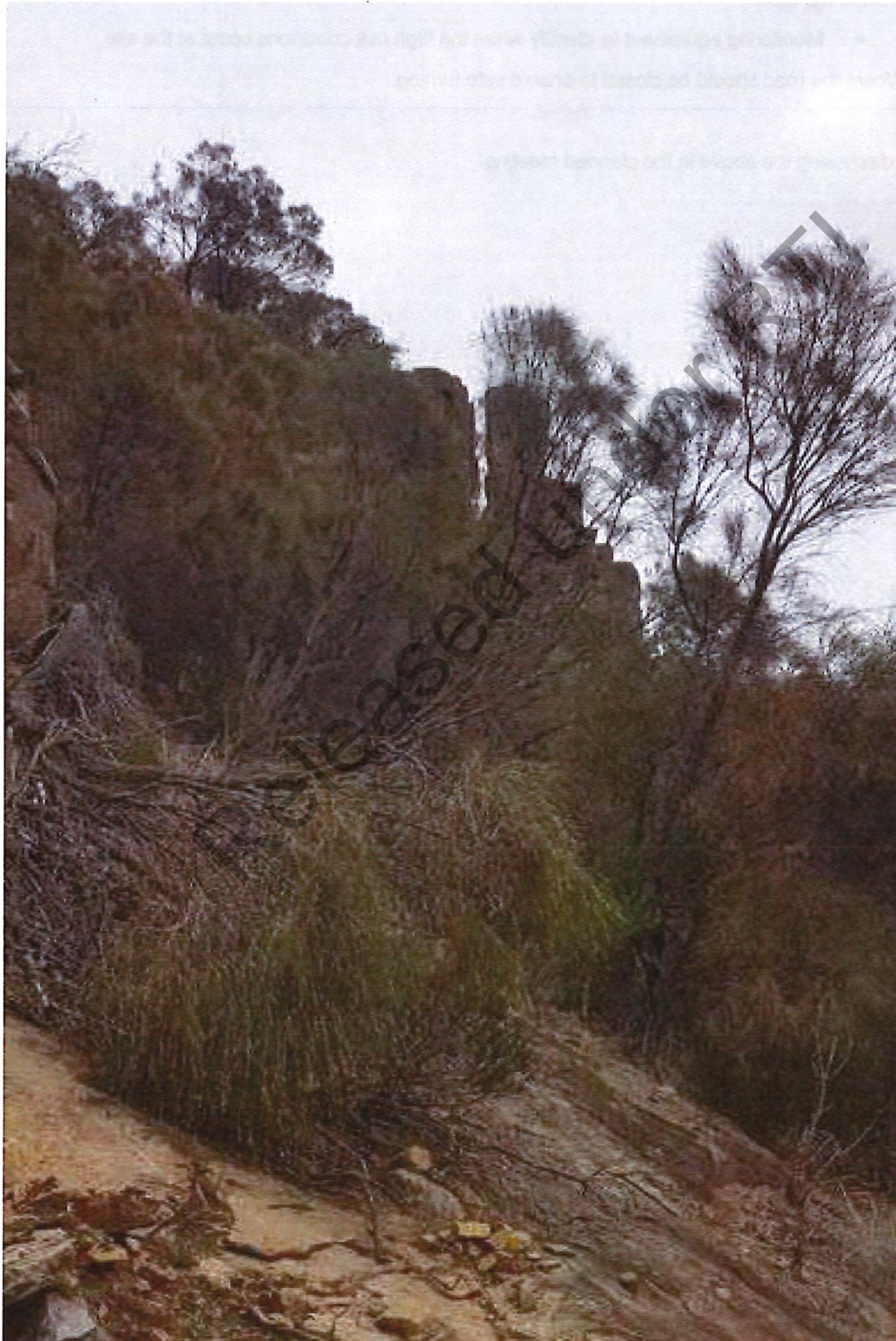
Figure 7: View of crack behind restrained boulder
