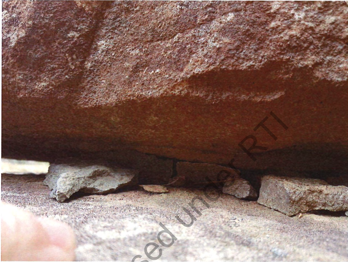
Figure 5: View under restrained boulder
