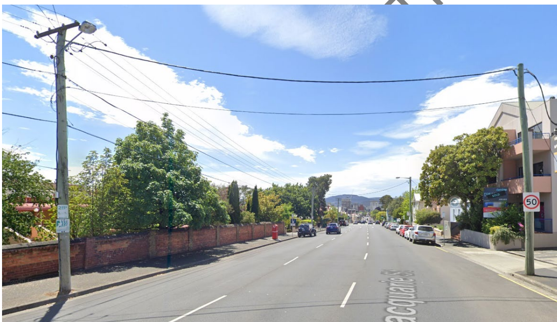
Figure 4 - Power poles at Back of Kerb Example
