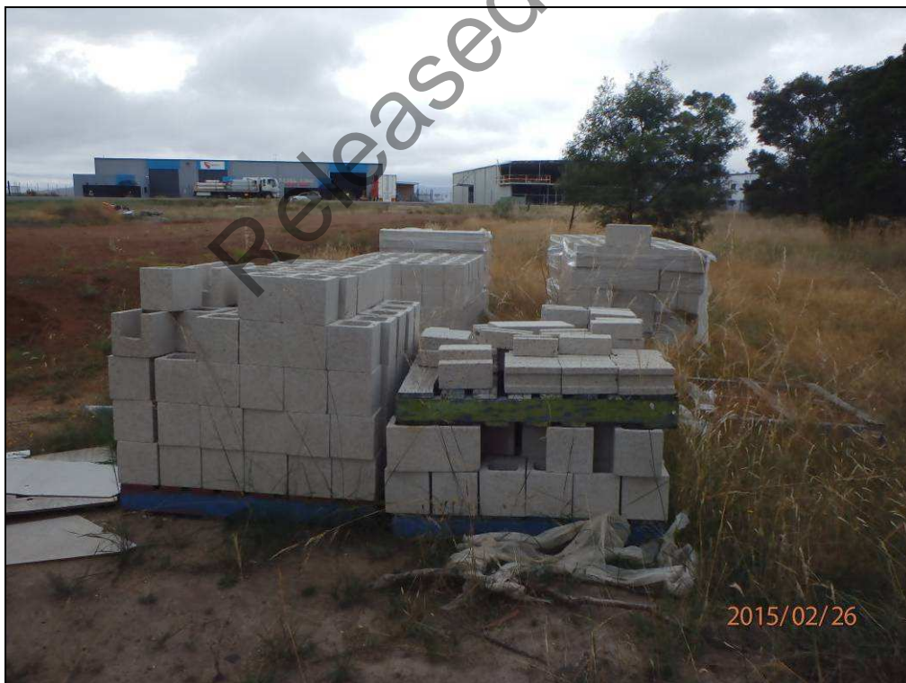
Building material being stored on site
