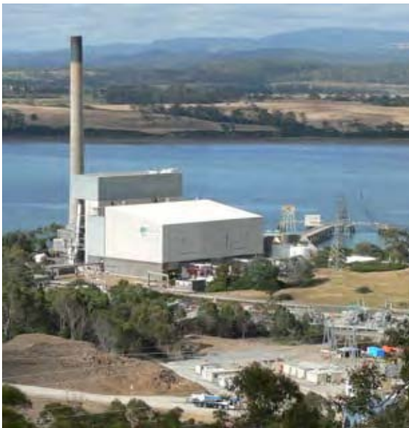
Bell Bay Power Station
