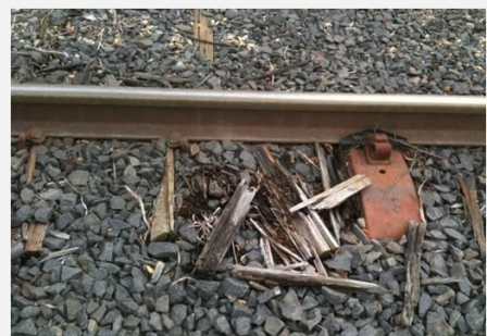
Photograph 3 – Condition of timber sleepers (source: Hyder, 2011)
