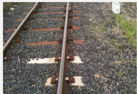
Photograph 2 – Combination of steel and concrete sleepers (source: Hyder 2011)
