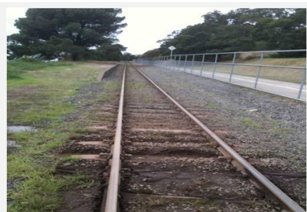
Photograph 4 – Track pumping (source: Hyder, 2011)
