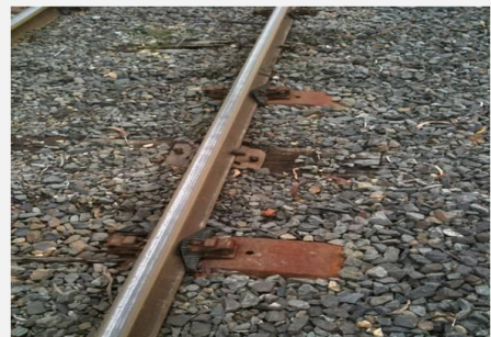
Photograph 1: Combination of timber and steel sleepers (source: Hyder 2011)
