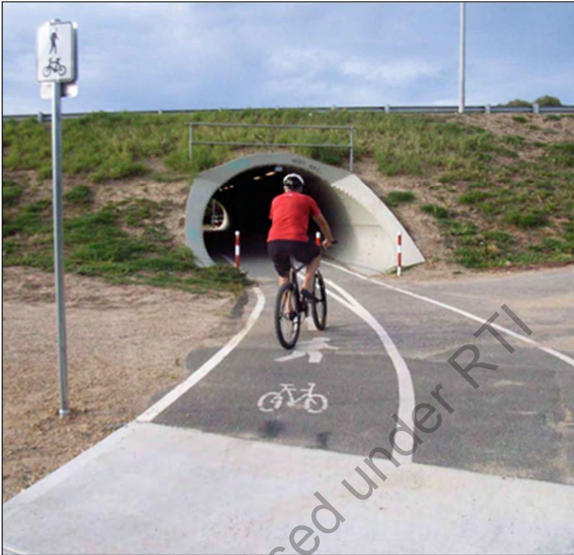
Figure 6 Off-road cycle path adjacent to a major highway, providing a bicycle route which is segregated from vehicle traffic
