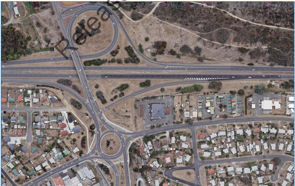
Figure 10: Junction of Tasman Highway and South Arm Highway, Mornington
