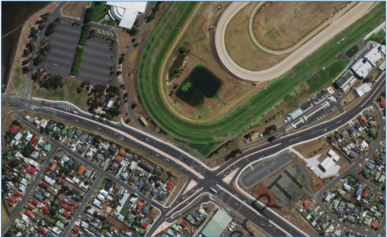
Figure 8: Brooker Highway and Goodwood Road intersection and adjacent areas
