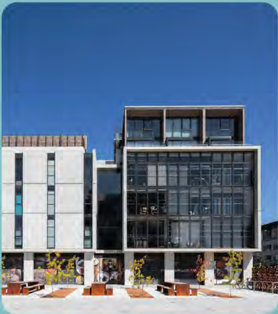
Cox Architecture for Chase Building Group Photography by Rodrigo Vargas
