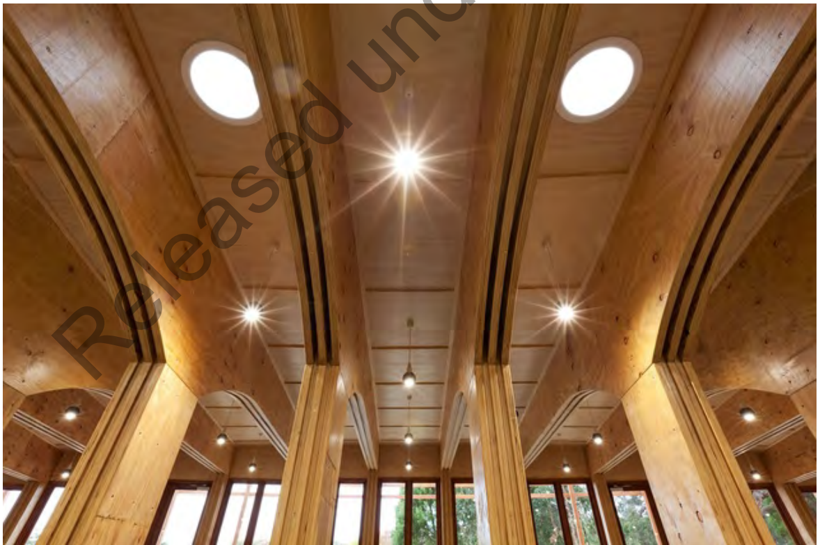
The ribs of the central resort hall, fabricated from layers of 5 ply sheets, glued into rigid frames.
