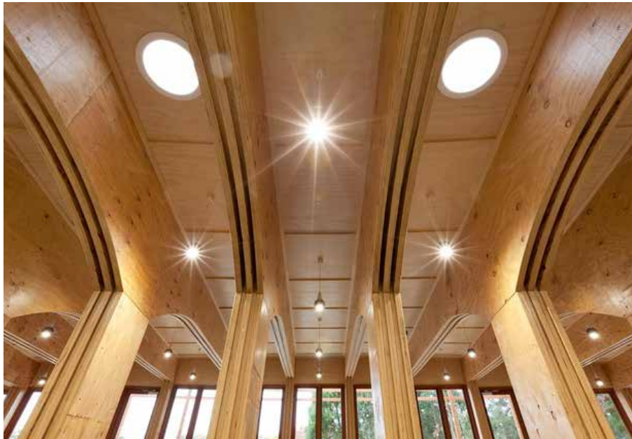
Laminated plywood to form the vaults
