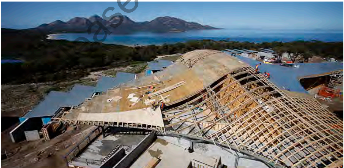
Saffire under construction by Fairbrother
