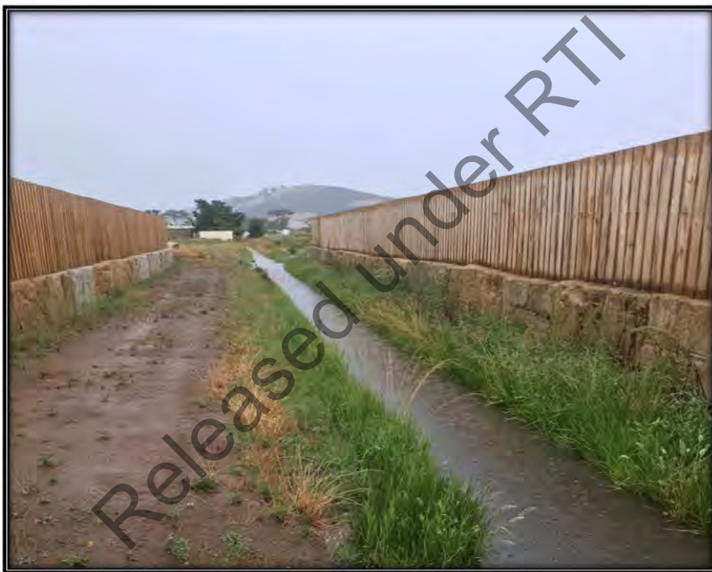
Figure 2 – Existing Sandstone stormwater channel and gravel access during rainfall event (Source: David Cundall, taken December 2021)
