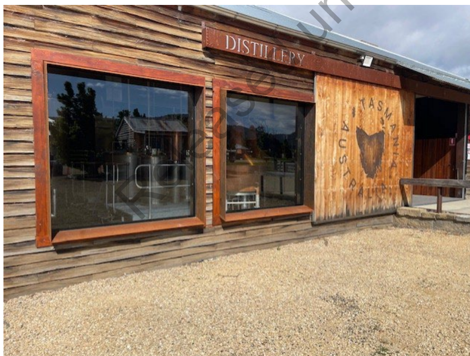
Windows giving view into restricted area
