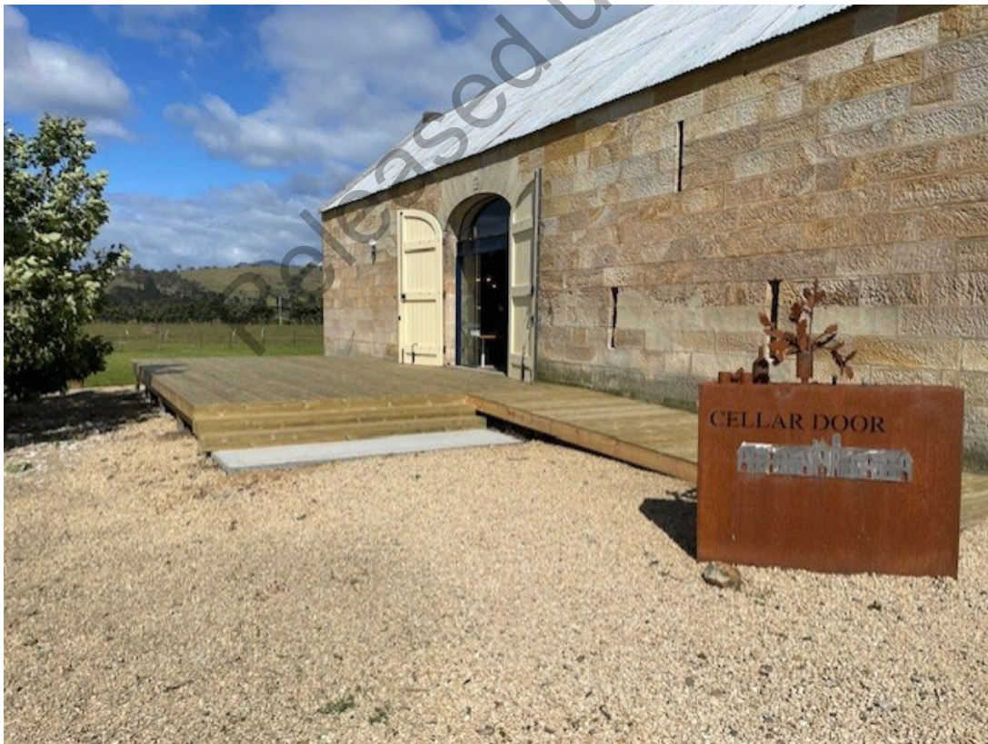
Decking supporting events and conference break outs (railing installed early Jan 2026)
