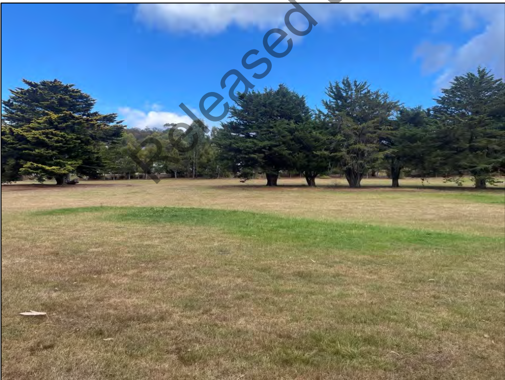
Figure 10 Green, lush grass potentially a sign of seepage
