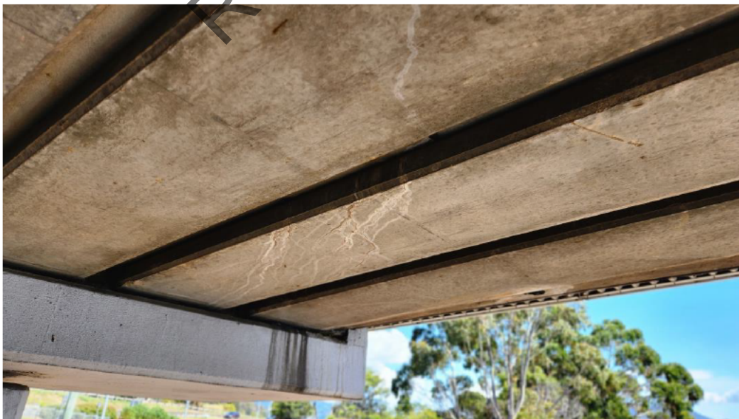
Figure 2 Cracking at second beam from the north between Piers D and E
