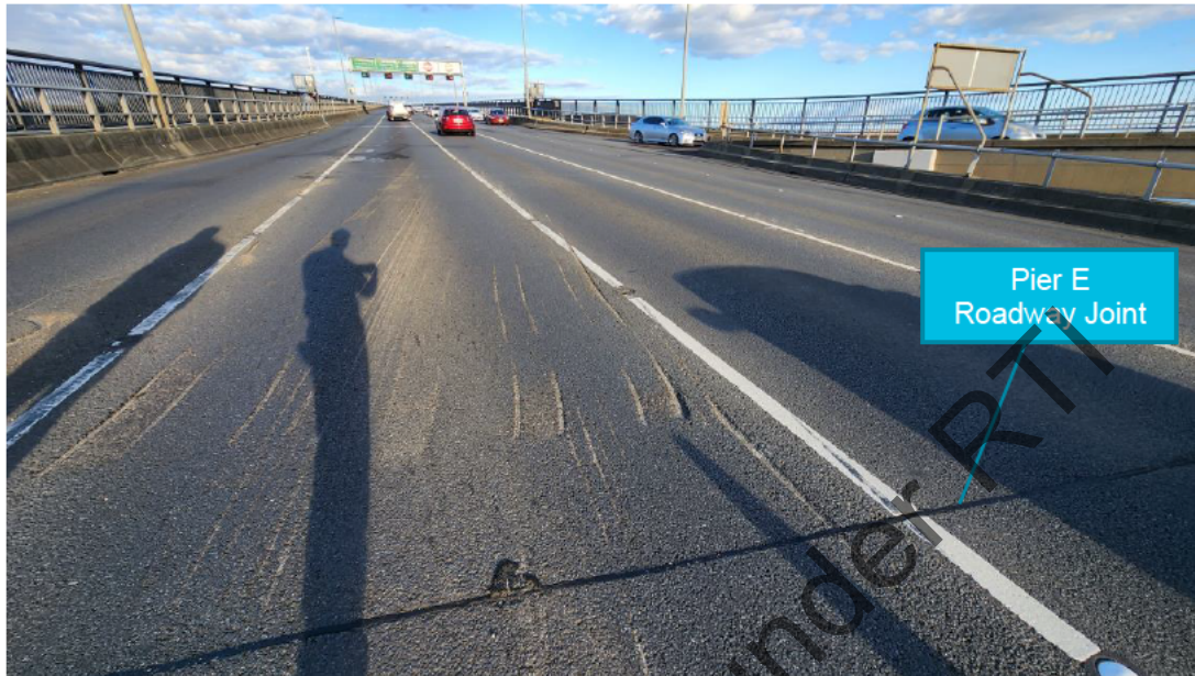
Figure 7 Gauges in the asphalt
