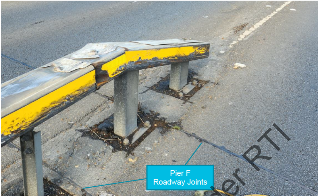
Figure 9 Cracking at the base of the barrier post
