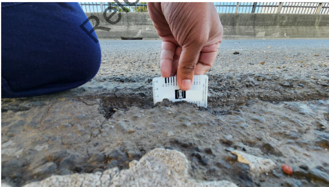
Figure 8 Depth of the gouges in asphalt
