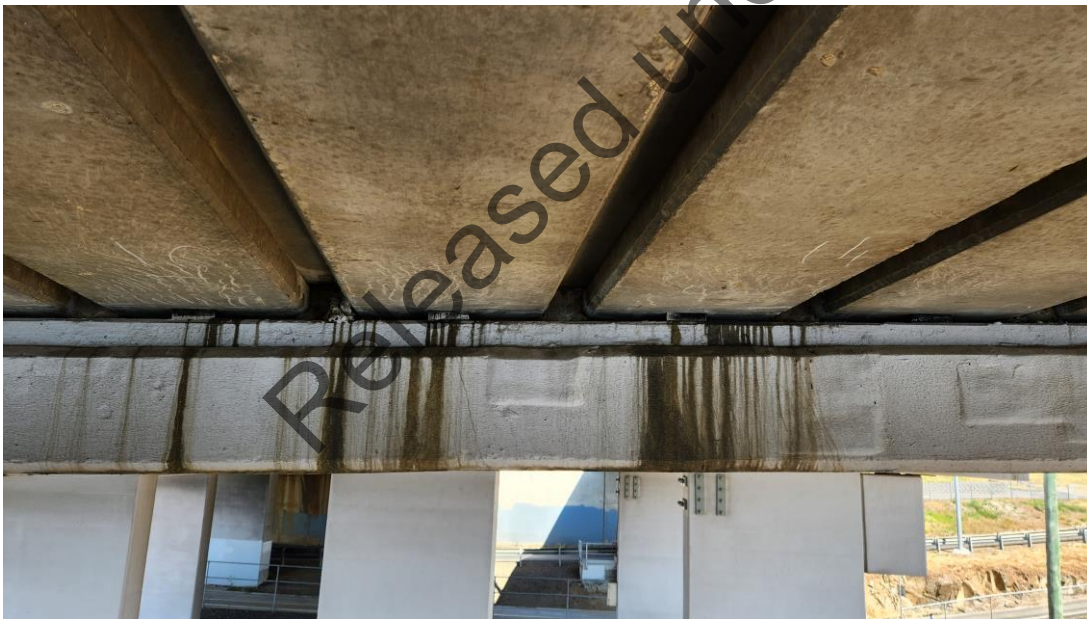
Figure 4 Staining on the eastern face of the headstock of Pier E
