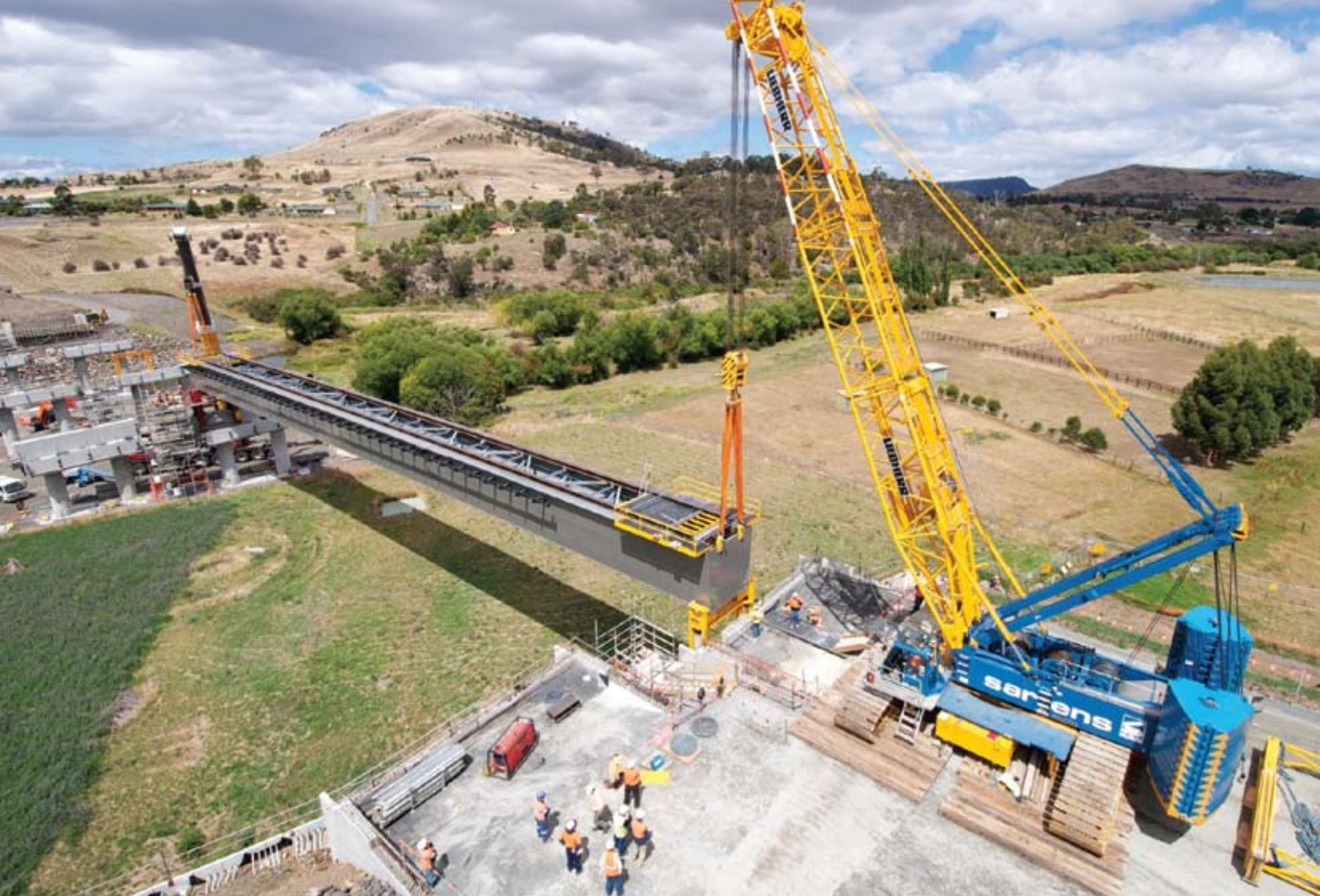
JORDAN BRIDGE UNDER CONSTRUCTION
